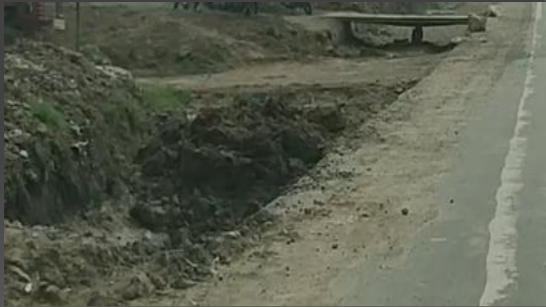
Figure 3: Construction activity along the road
